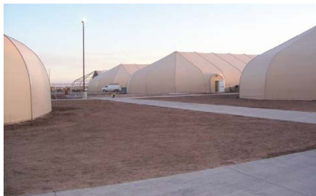
Dormitories constructed from steel beams covered by tough canvas like water proof fabric. AKA - SPRUNG structure
